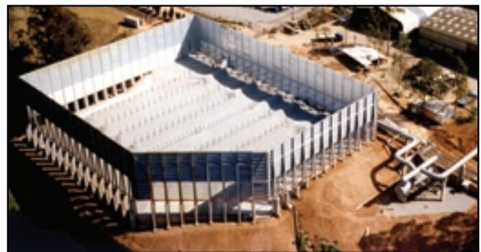
*The LRGO multi-burner flare system can be provided with radiation fences that completely shield the flame visibility and radiation at grade.*
