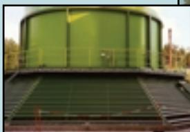
*The natural draft design of the KEGF flare provides non-assisted, smokeless, non-visible flaring in a cost-effective enclosure design.*
