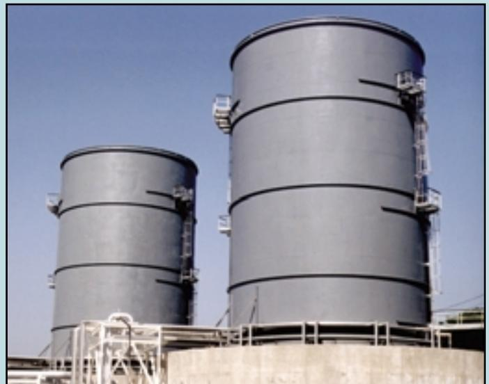
*The ZTOF flare design has been used to provide up to 200 ton/hr enclosed flare capacity in a dual unit enclosure design.*
