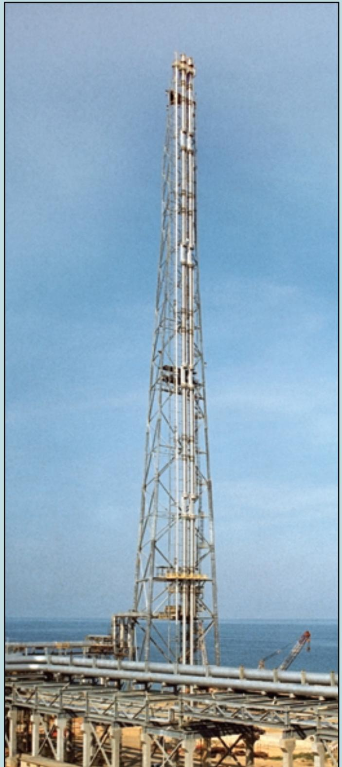
John Zink's demountable derrick structures allow multiple flares to be installed on a common structure. The demountable design allows the individual flare tips to be lowered to grade while the other flares remain safely in service.
